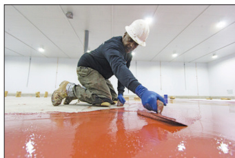
Roland King, with Surface Technology Inc., spreads urethane mortar onto the floor of a food processing facility. King is a 20-years employee of the Manheim Township-based industrial flooring contractor. PHOTO/AMY SPANGLER
